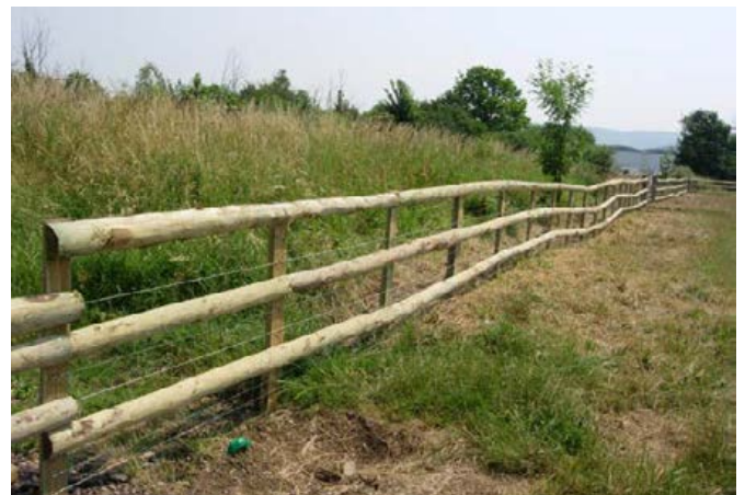
Timber post and rail fencing
